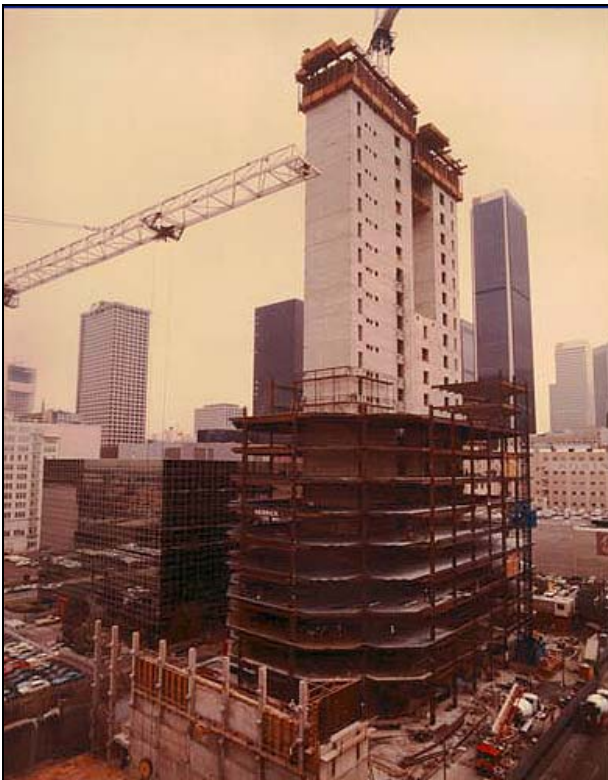
Jump Form In Use -utilizes crane and bucket for concrete pour
